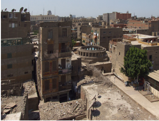
Figure 142) Three different states of conservation evident: on the left hand a BAD state, in the foreground a GOOD state and in the background the DILAPIDATED roof of a former hammam, whose dome has collapsed.
