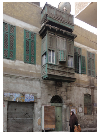
..... Figure 152a, 152b) A building in a FAIR state of conservation has achieved fair scores overall in the previous sections. The structure of the building is sound, but some problems might exist in a mild form only, such as erosion, water stains or minor cracking.
