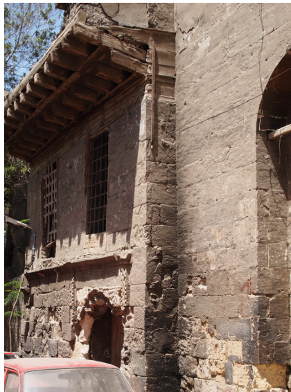
Figure 130a, 130b) Two examples of stone walls intentionally built to have the same stones exposed as a finish.
