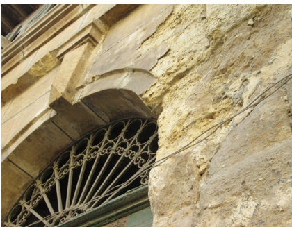
..... Figure 258) Stone erosion indicates a structural problem, Haret al-Dohedira, Sayeda Zeinab.
