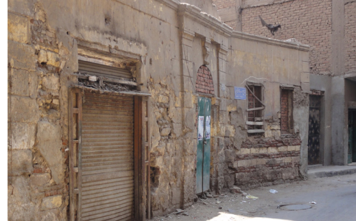
Figure 142a, 142b) A LIGHT BULGING is the beginning of a consistent one ; it is slightly visible and can occur both to buildings (due to structural failure or excessive vertical pressure) or to ruins, such as in the left figure. In this case, the bulging is probably caused by the pressure of the inner solid waste load and lack of horizontal supports.
