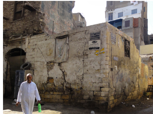
Figure 137) A DILAPIDATED finish is so damaged that it has almost disappeared entirely.
