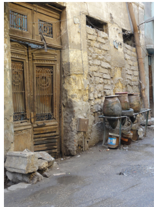
Figure 143a, 143b) A HEAVY BULGING is a visible deformation in the lower part of a wall, either close to the ground or – in the case of upper floors - closer to the horizontal supports.
