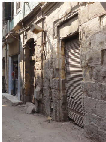
Figure 150a, 150b) Heavy erosion affecting the stone structure and destroying mouldings and decorative elements.
