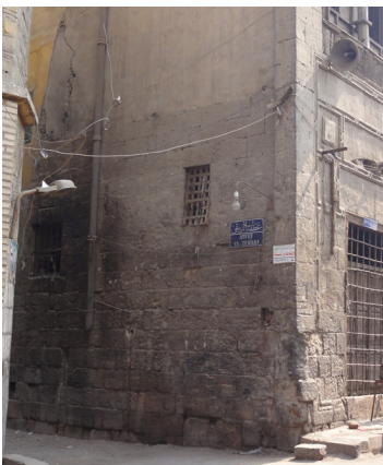
..... Figure 145) A MEDIUM CRACK PATTERN presents random cracks that do not affect the majority of the façade but are of a consistent thickness.
