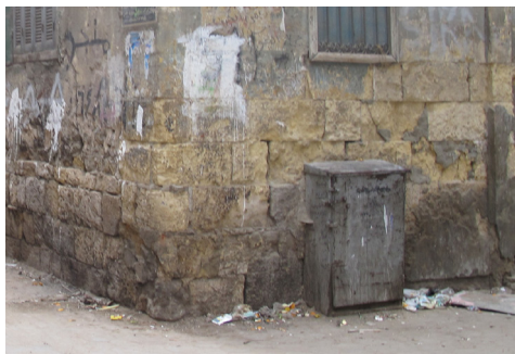
..... Figure 211) Electricity substation installed in the street.
