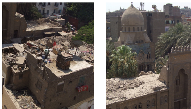
..... Figure 141a, 141b) Two roofs in a BAD state of conservation: displaying lack of structural integrity, overloading and weaknesses.
