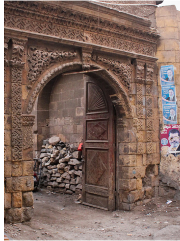
Figure 149a, 149b) Two cases of light erosion due to mechanical impact and lack of maintenance, as well as water infiltration problems (right side).
