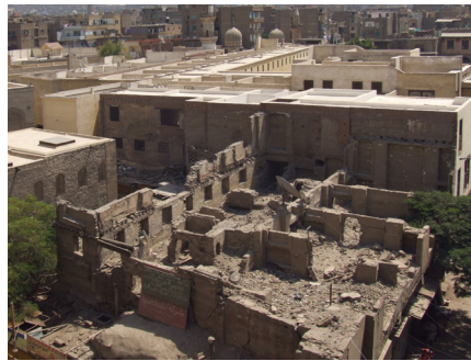
Figure 141a, 141b) A DILAPIDATED roof is a partially collapsed roof that has completely lost its structural integrity and can no longer be maintained.
