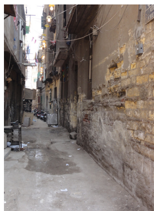
Figure 148a, 148b) Two cases of major water stains that have seriously damaged and eroded the materials in the lower part of the facade.
