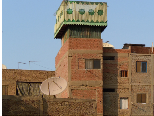
Figure 129a, 129b) The absence of a finish exposes the structure to the elements, increasing potential risk of damage and having unpleasant visual results. The exposed structure may be of any kind of material.
