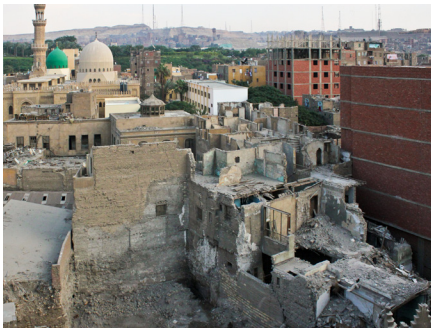
Figure 141a, 141b) A DILAPIDATED roof is a partially collapsed roof that has completely lost its structural integrity and can no longer be maintained.
