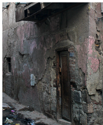
..... Figure 146a, 146b) A HEAVY CRACK PATTERN is a serious structural condition where cracks are severe due to their size, location, depth and diffusion.
