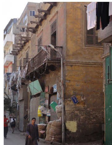
..... Figure 123) A structurally sound building but with minor damage: FAIR state of conservation for the structure because of ground floor erosion of stones and minor superficial crack patterns.
