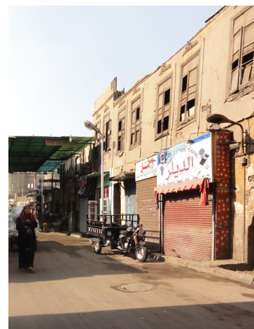
..... Figure 124) A building whose structure presents some signs of failure: BAD state of conservation for the structure because of bulging walls to the upper floor.
