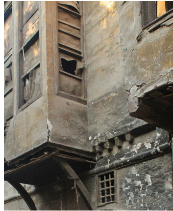
..... Figure 144a, 144b) A LIGHT CRACK PATTERN presents random, superficial cracks that do not affect the majority of the façade and are not located in dangerous areas, where they might threaten the building's structural integrity (e.g. corners of openings, corners in general or lintels).
