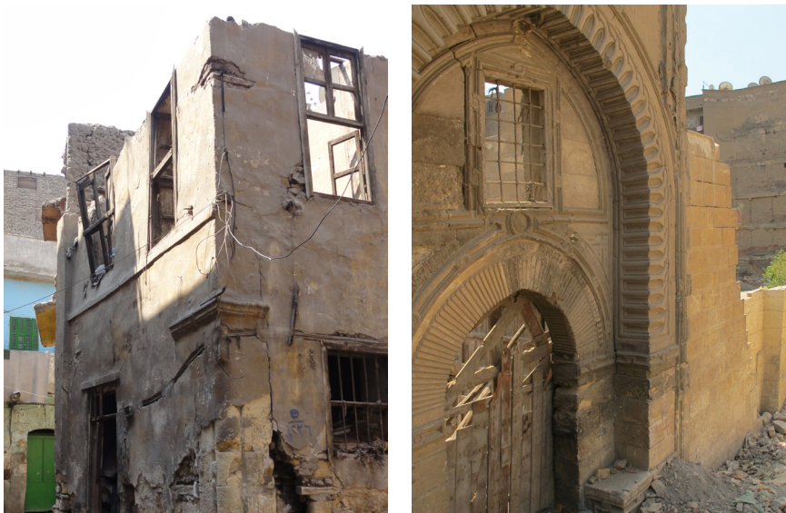
Figure 138) Two cases of visible roof collapse and absence.
