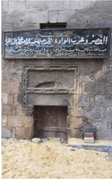
Fig. 015: Wooden sign in a bad condition, it is not a heritage sign but it is a sign of the building tenant, NGO of social development, there is no mention of the monument name nor function. And the sign is fixed inappropriately hides behind it architecture elements and a window on the facade. URHC photo-bank
