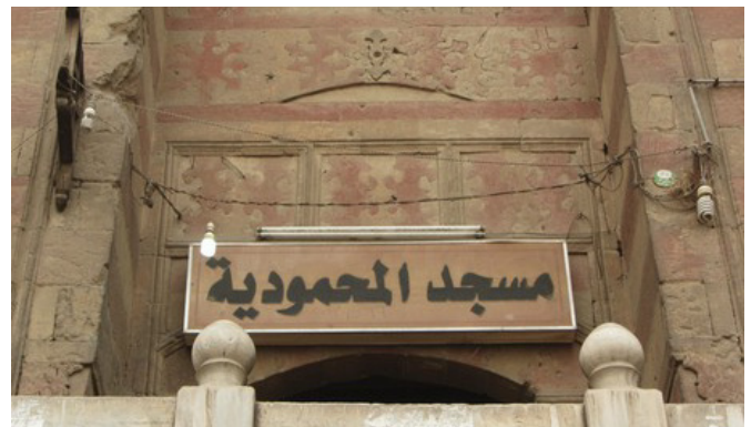
Fig.71g: El-Mahmoudeya Mosque, a self-illuminating sign stating only the monument name. Its inappropriate design and location disfigure the entrance and its architectural features
