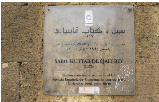
Fig.71c Sabil Kuttab Qait-Bey. Plaque contains information on the listing number, dates of construction and restoration done by the Spanish Agency for International Development Cooperation. The plaque in Plexiglas is not easy to maintain with the dust of Cairo and shows signs of a lack of maintenance
